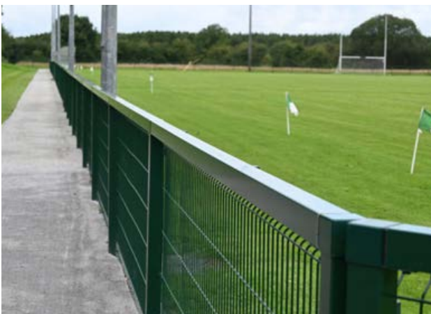
Ballyfore GAA - completed fence.
